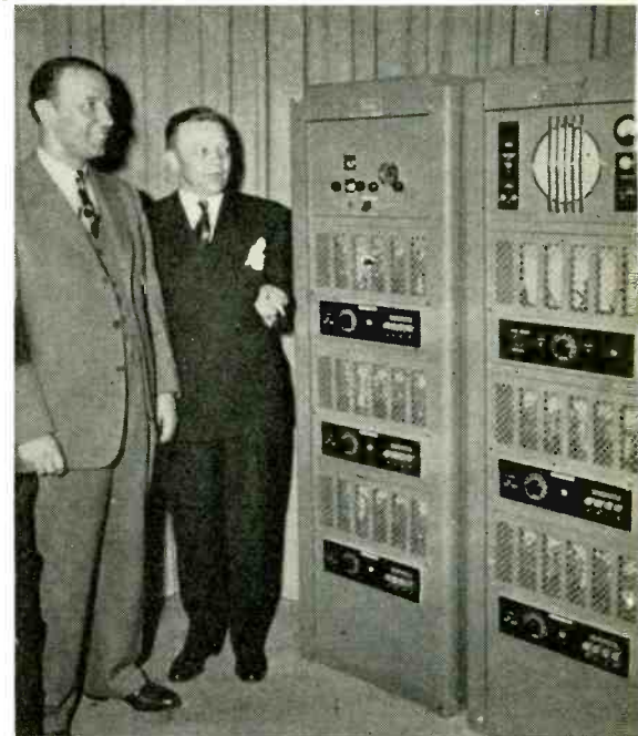
Ralph Walker and Arch Samuelson inspect the Operadio "Plant-Broadcaster" installation which provides music, work-paging and personnel announcements through 131 loudspeakers in the Johnson & Johnson plant in Chicago.
